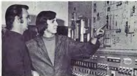
Maintenance electricians John Blything, left, and Chris Roberts on duty at Five Fords.
