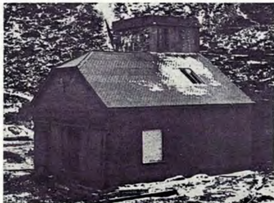
The original No. 1 Transformer Station . . .
